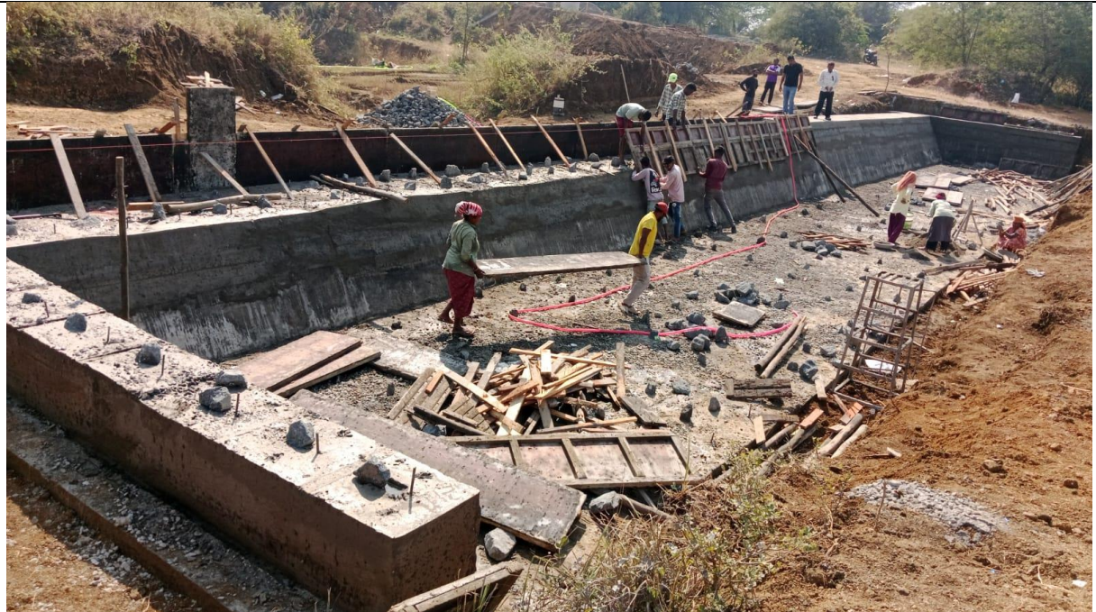
Checkdam construction at Waliya Block, Bharuch district, Gujarat
