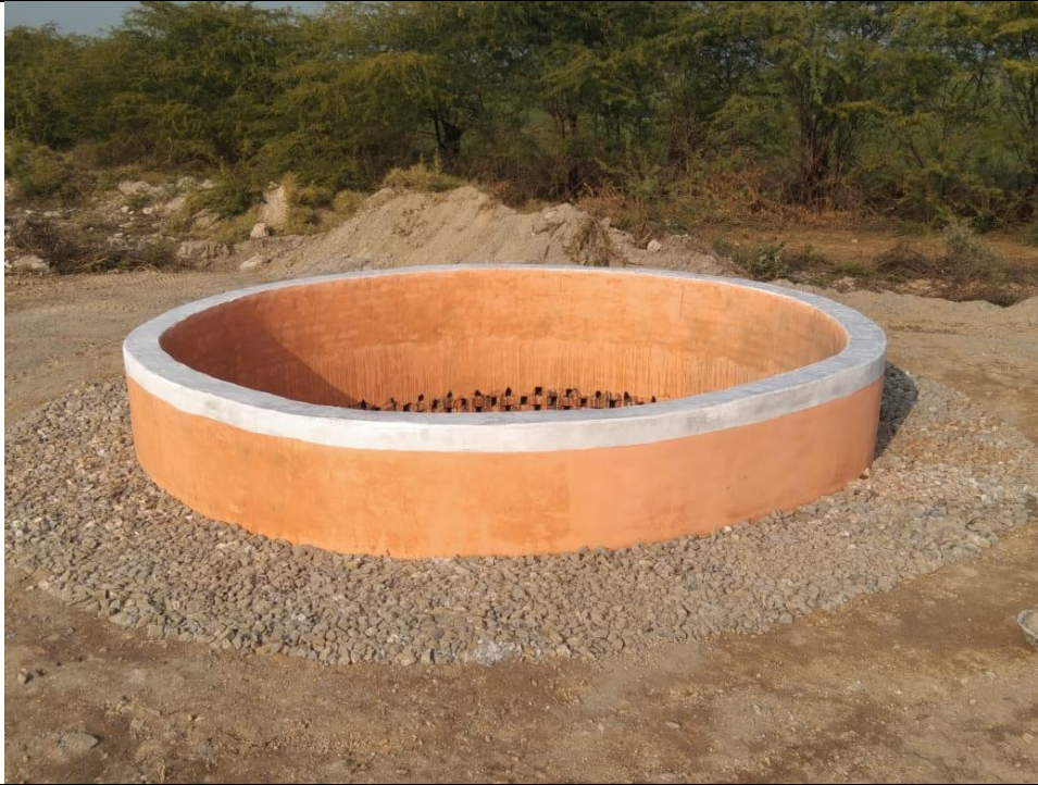
Ground Water Recharging Well "Khambati Kua" – Dudu Block, Jaipur
